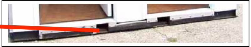
Fig. 2 - Tine Ports (Steel Frame)
